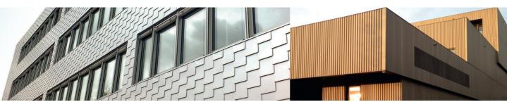
**hm-eloflex**<sup>®</sup> is an innovative form of modern coil anodizing. The metallic surface created by this processing allows the material to be reshaped without significant impairment of the anodized layer.
