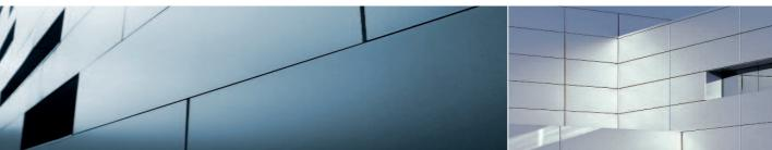
hm-falzit® structur coloured aluminium in double standing seam quality is a rolled aluminium product that is coil-coated with a textured paint.
