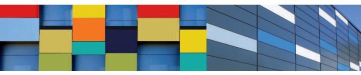
**ProColoR=t** coloured aluminium is a rolled aluminium product which is polyester powder-coated using coil coating technology.
